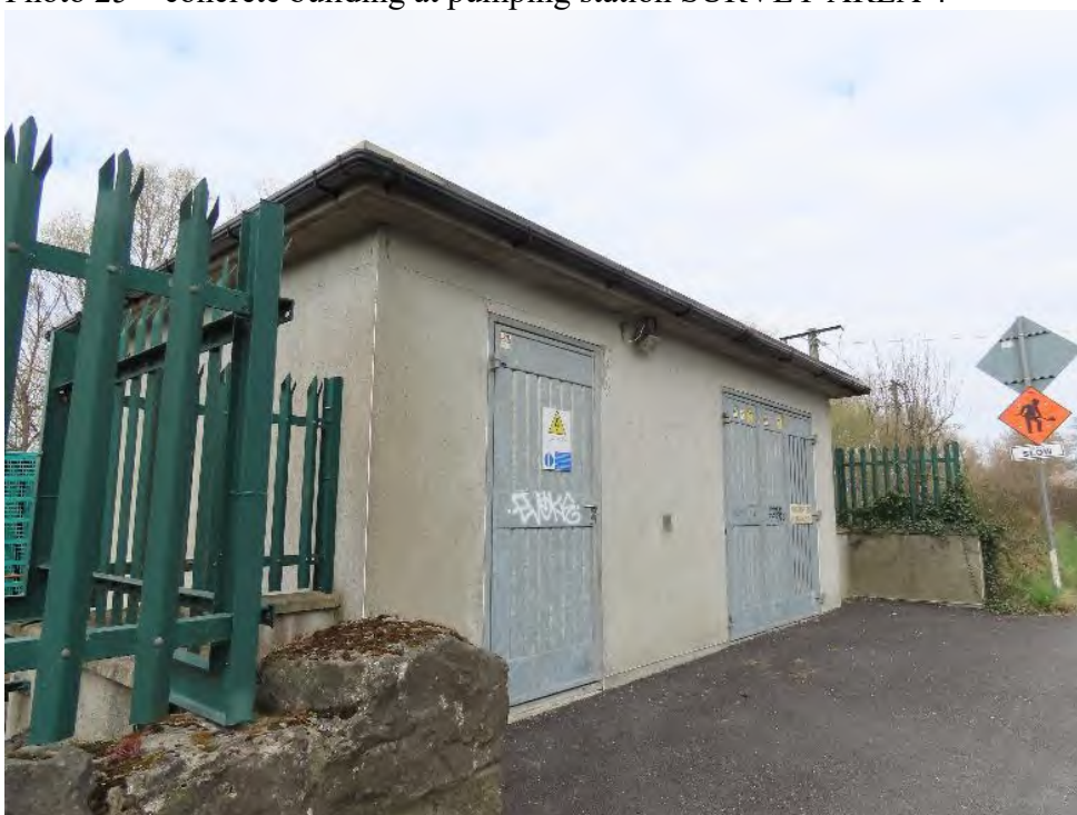
Photo 26 - concrete building at pumping station SURVEY AREA 4
