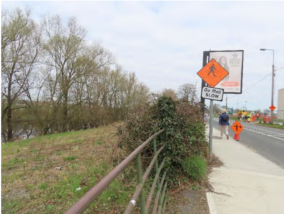
Photo 27 – area to north of pumping station between R448 and River Barrow
