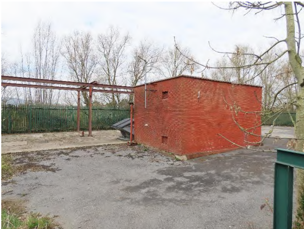
Photo 24 – red brick building at pumping station SURVEY AREA 4
