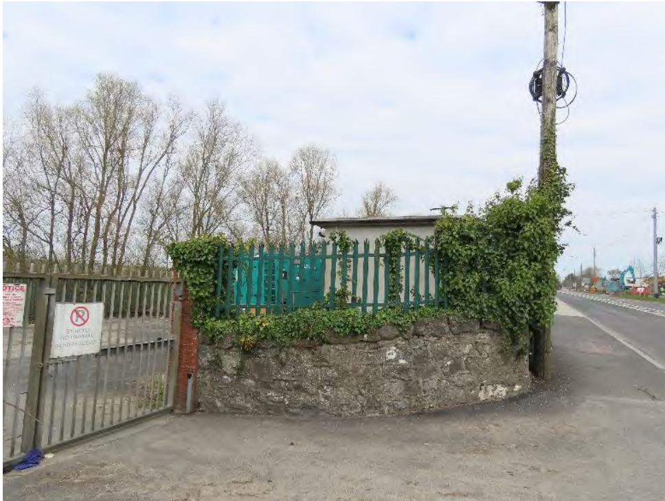
Photo 25 – concrete building at pumping station SURVEY AREA 4
