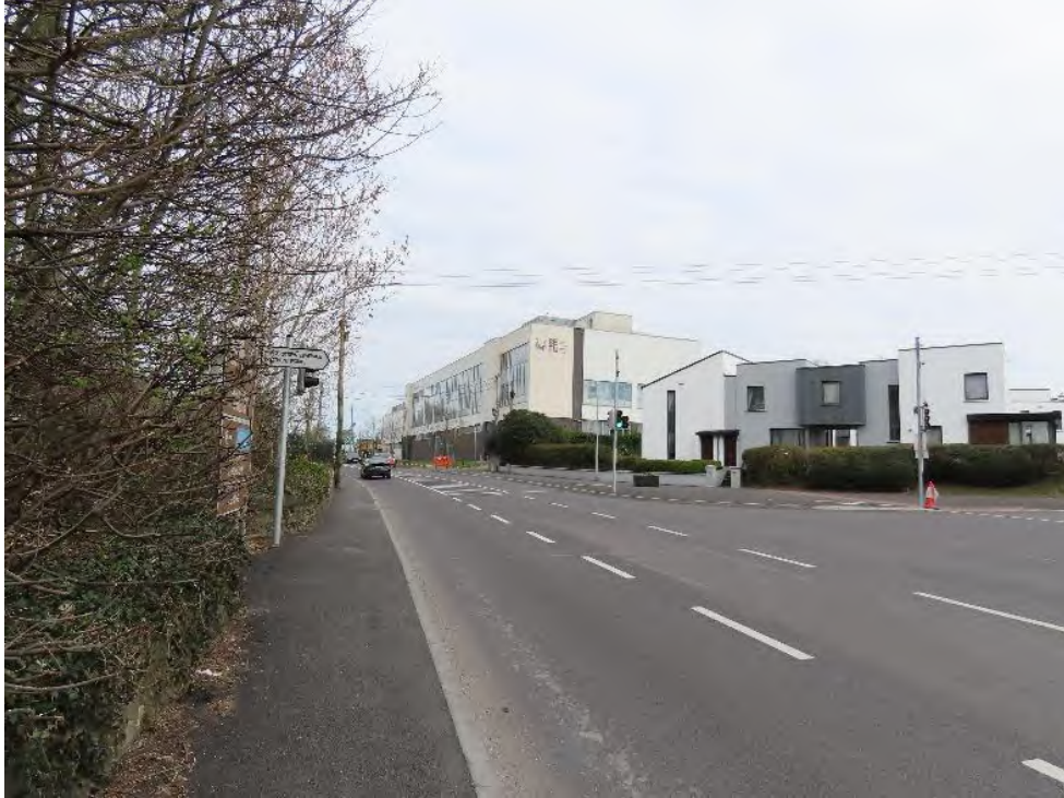
Photo 23 – looking north towards South East Technical University building
