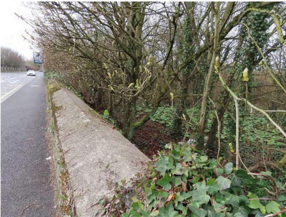
Photo 30 - wooded area to south of pumping station
