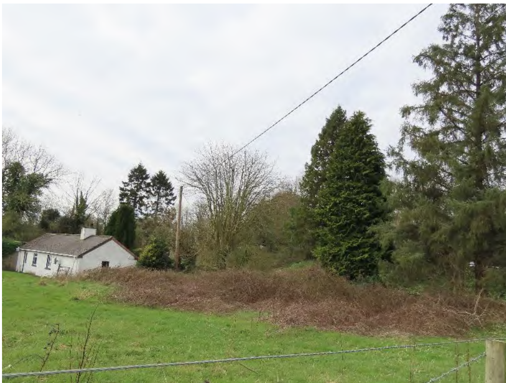
Photo 6 - rear elevation and northern gable of cottage. SURVEY AREA 1
